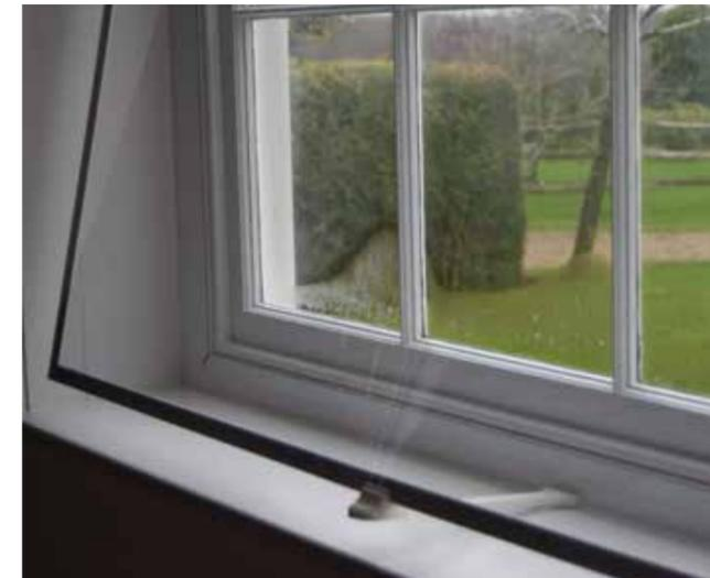
The two test windows with WindowSkins in position. The line of the magnetic strips can just be seen around the perimeter of the windows
