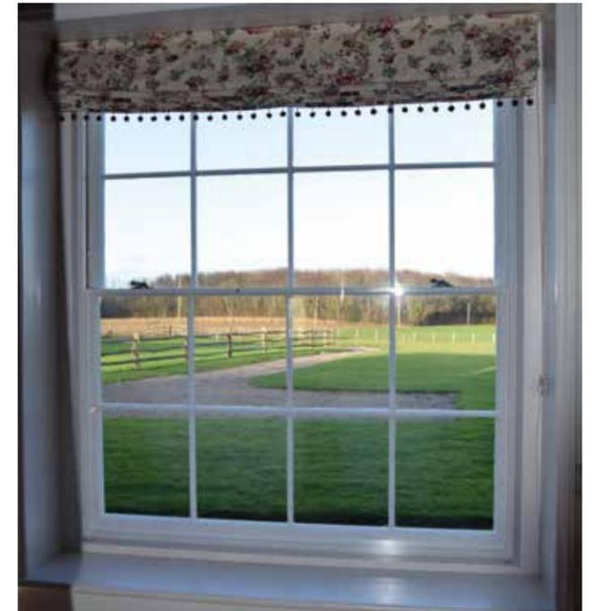
On the two windows tested, drafts were stopped and condensation problems were reduced to a light misting on the colder winter mornings. On the smaller of the two test windows light condensation occasionally appeared on the room-side surface of the WindowSkin but it was quickly removed with a single wipe of a cloth.
